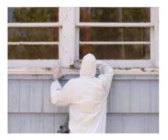
Lead-based paints were banned for residential use in 1978. However, homes built before this time most likely still contain some level of lead-based paint. When this paint peels and cracks, lead paint chips and dust forms. Surfaces covered with the lead-based paint where paint might wear by rubbing or friction can cause lead dust. This includes locations such as windows, doors, stairways,
